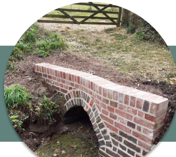
Cart bridge at Bere Mill on the Upper Test after restoration in 2021 © Kathryn Boler
