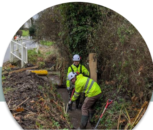
Wessex Rivers Trust staff digging out a sediment ditch on the Cheriton Stream in 2025 © Wessex Rivers Trust
