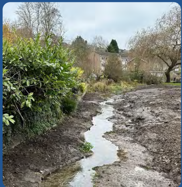
Example of after De-canalising, Chesham Moor
