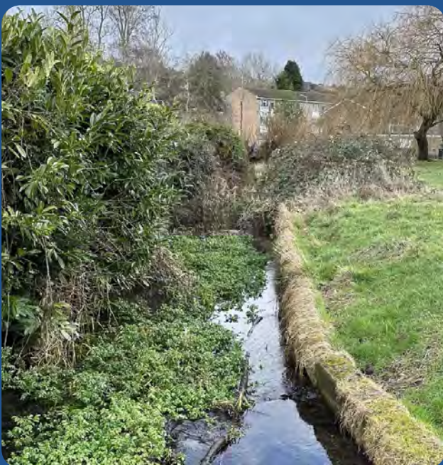
Example of before De-canalising, Chesham Moor
