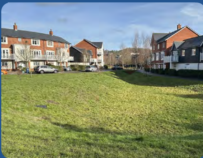
SuDS at Wye Dene Estate, High Wycombe
