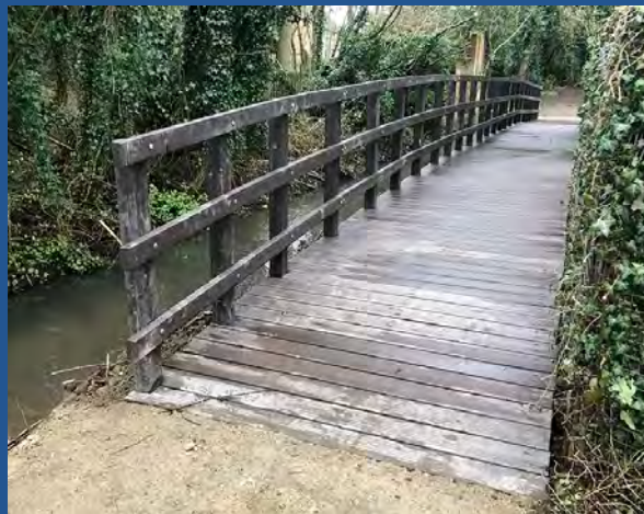
Boardwalk - Meades Water Gardens, Chesham
