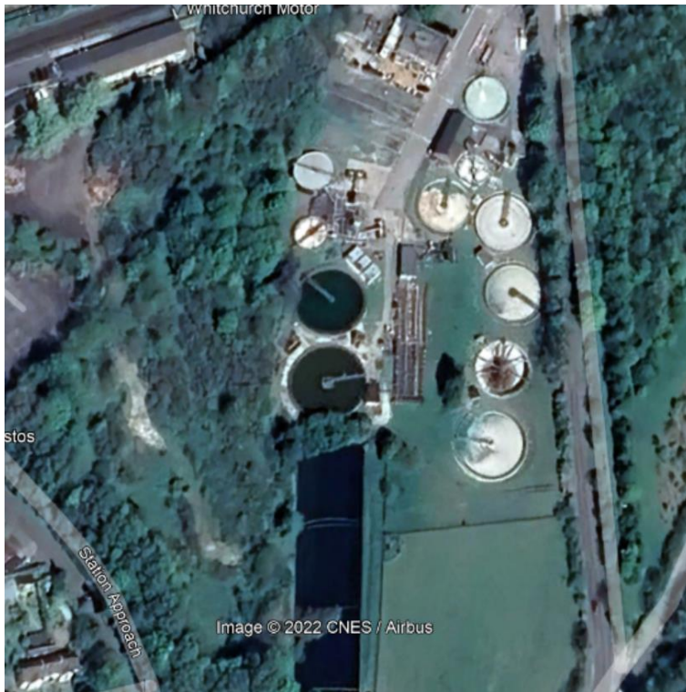
Figure B17 Aerial image of Portals WWTW dated April 2022
