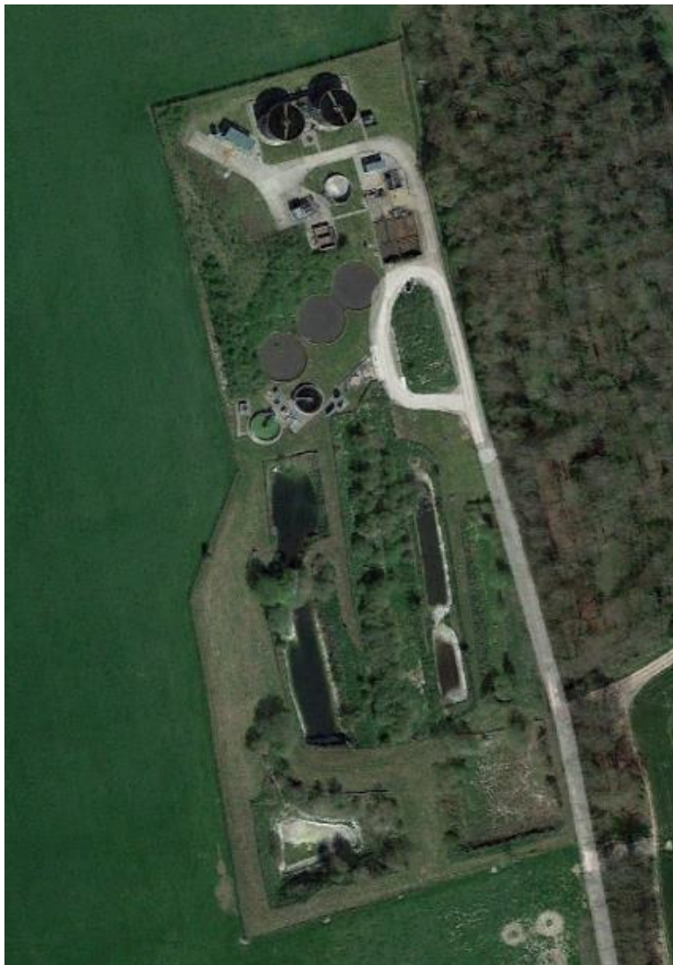
Figure B12 Overton WWTW in 2017
