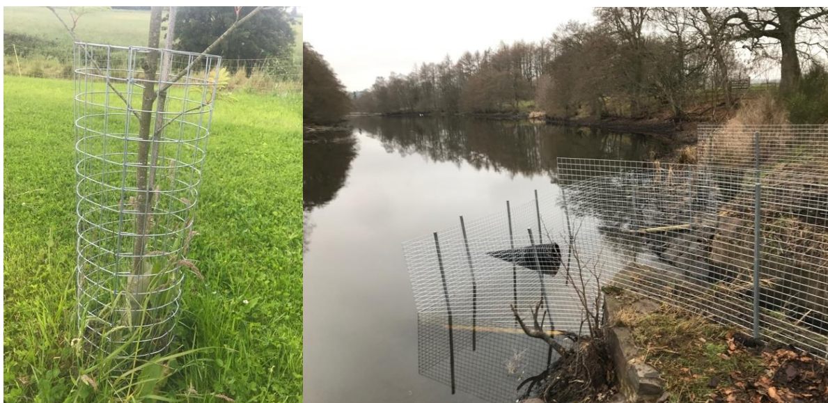
Figure 29. Examples of Scottish beaver mitigation including a fence-wrapped tree, and a flow device structure protecting a culvert.
