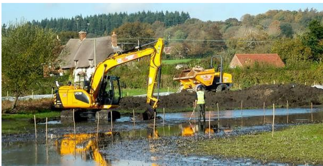
Figure 82: Excavation of Round Pond during 2014 (Photograph: Jo Gore).
