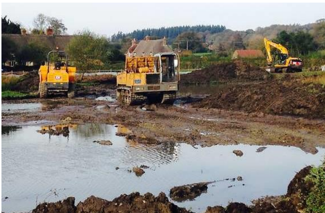
Figure 83: Excavation of Round Pond during 2014 (Photograph: Jo Gore).
