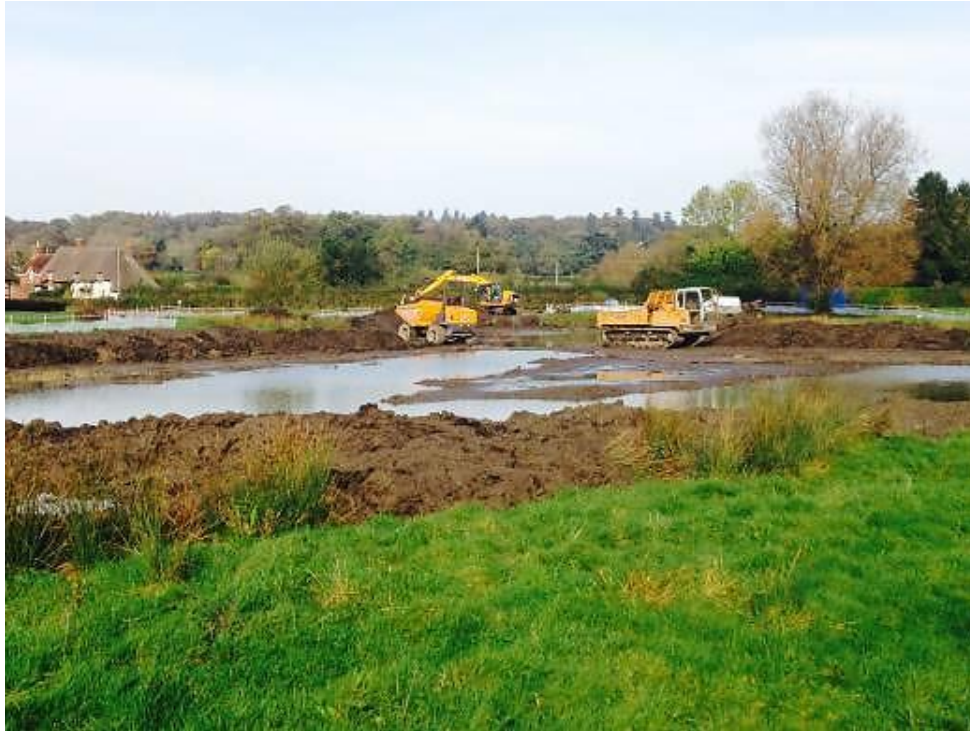
Figure 84: Excavation of Round Pond during 2014 (Photograph: Jo Gore).
