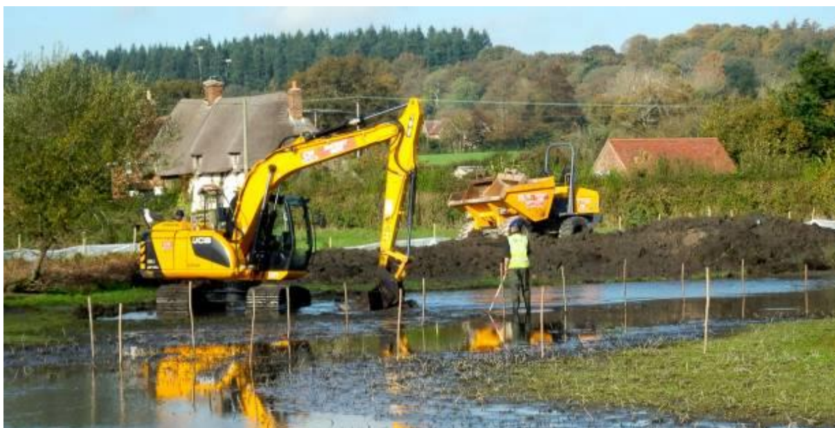
Figure 7: Excavation of Round Pond during Autumn 2014
