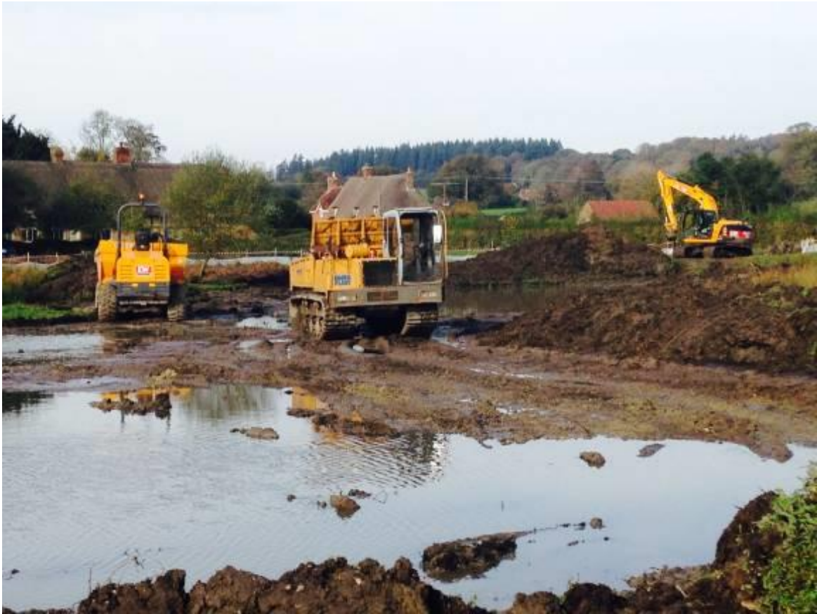
Figure 8: Excavation of Round Pond during Autumn 2014
