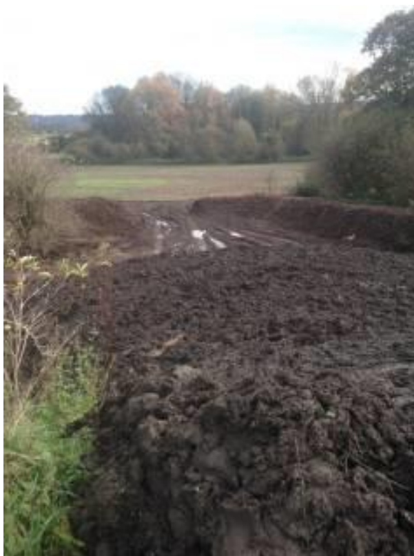
Figure 11: Material in hollow before bund was closed
