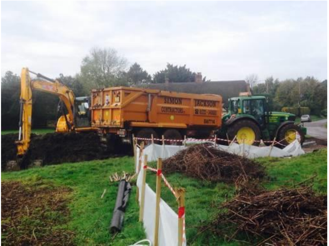
Figure 10: Excavation of Round Pond during Autumn 2014
