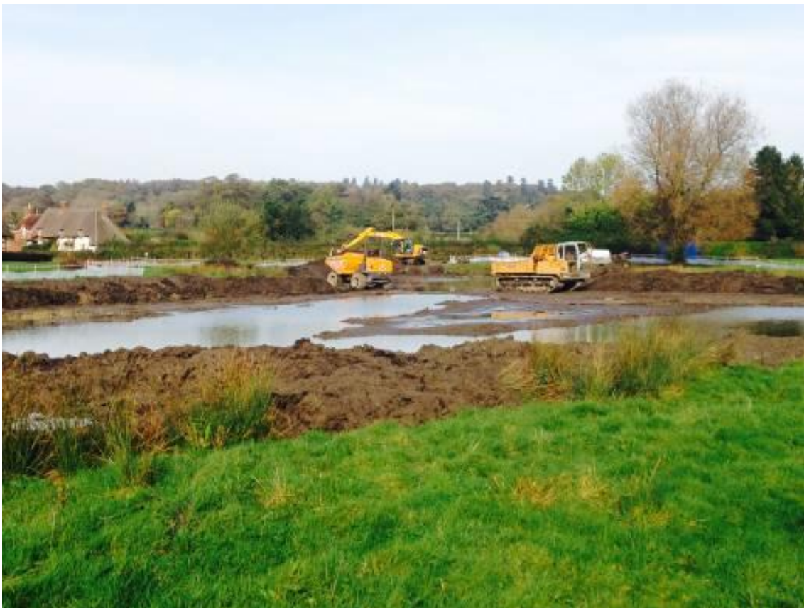
Figure 9: Excavation of Round Pond during Autumn 2014
